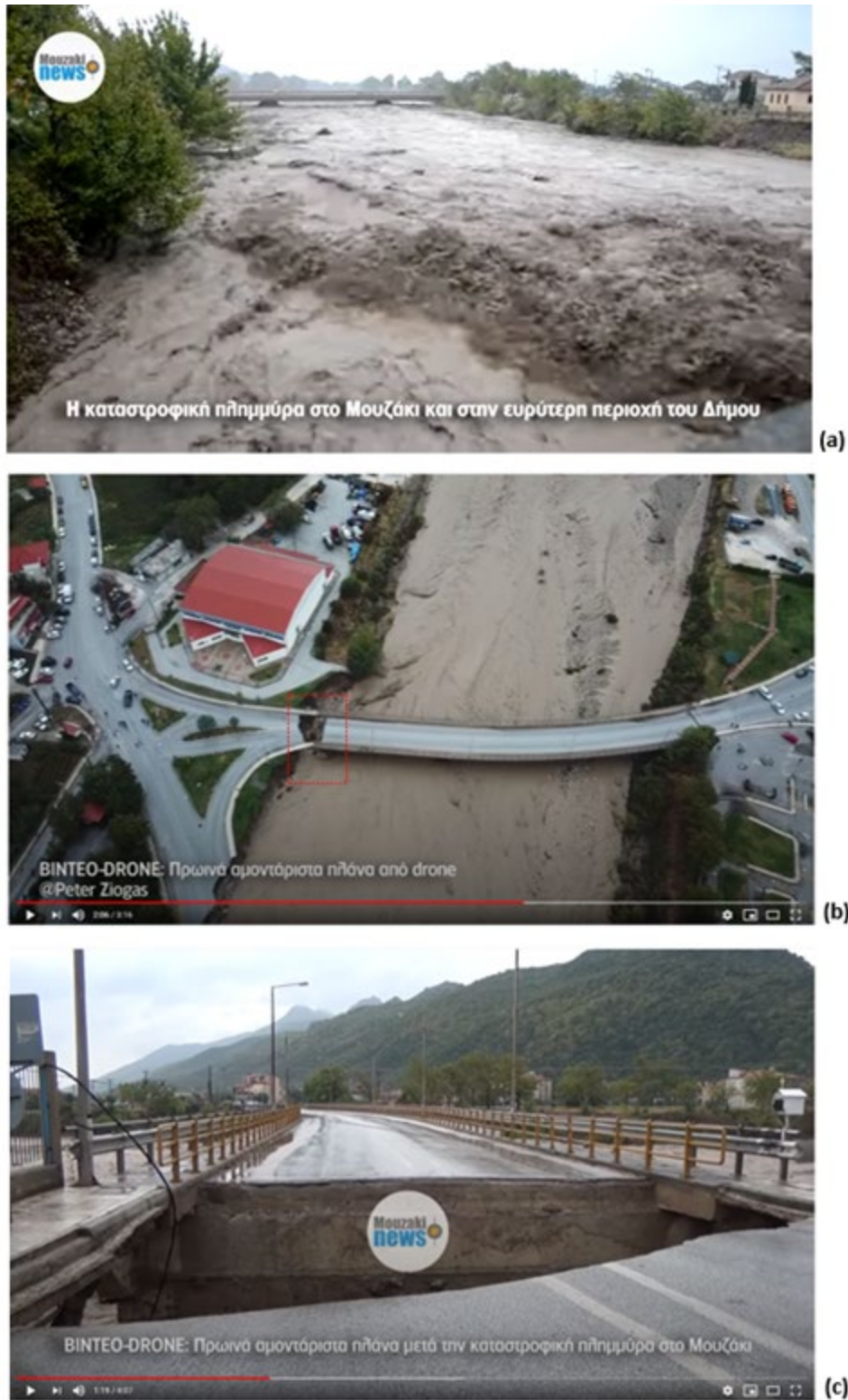
Figure 5.16. Footage of Bridge No. 7, in local news showing: (a) the water height on September 18, 2020 ( https://www.youtube.com/watch?v=7TzUZh3YgxY ); and (b) – (c) the abutment failure and associated roadway collapse ( https://www.youtube.com/watch?v=hLP3NdMF9SI ).
