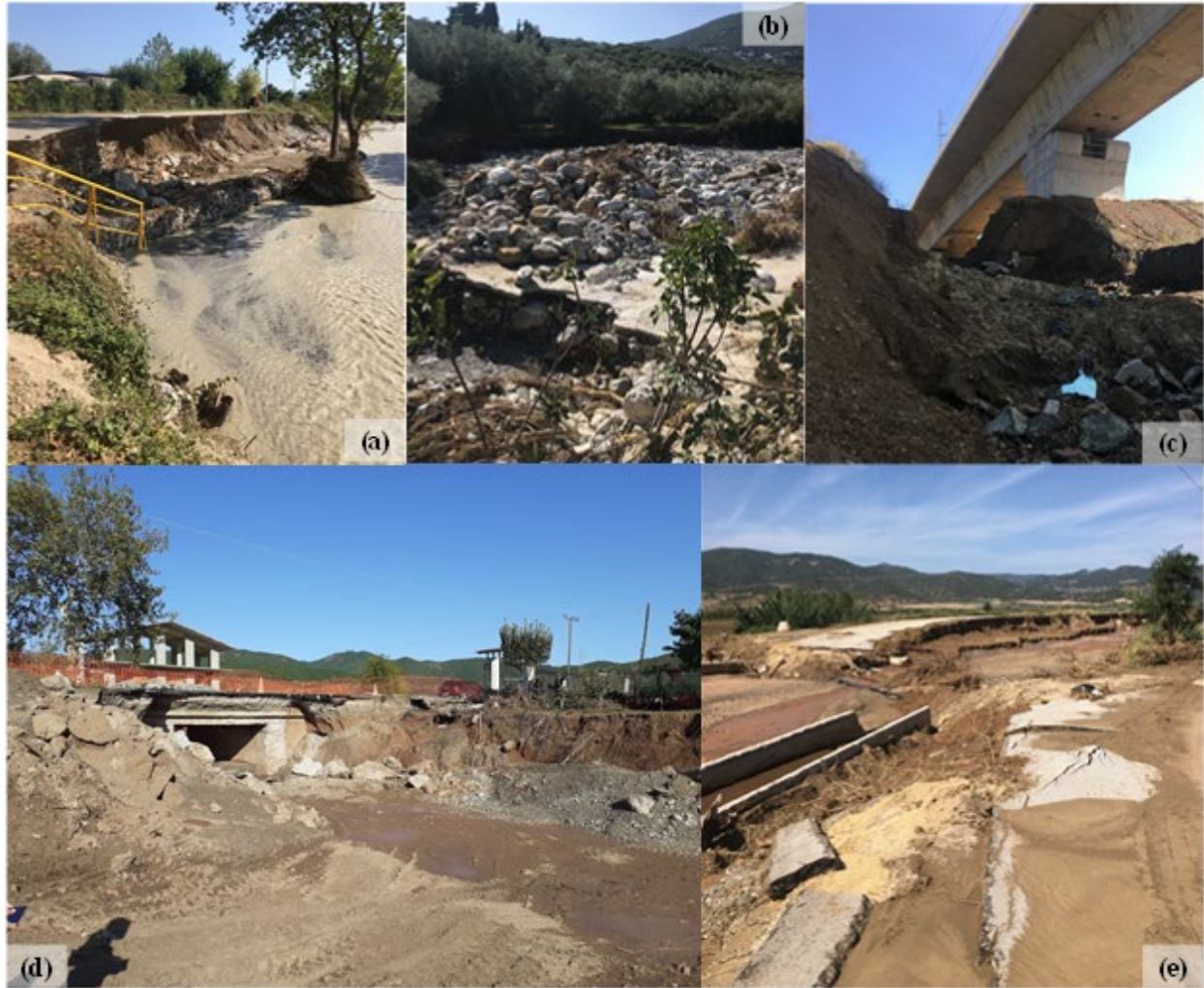
Figure 4.14. Characteristic damages in the region of Lamia following Medicanne Ianos: a) riverbank erosion and road embankment failure, b) extensive debris flow, c) bridge foundation scour, d) riverbank erosion, and e) road embankment failure
