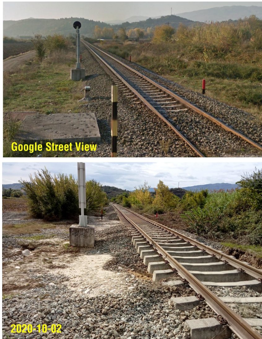
Figure 5.41. Railway embankment & ballast scouring along Paleofarsalos-Kalabaka line, near Magoula (39.45127°N, 21.78824°E). Comparison of field photo (bottom) with pre-event Google Street View image (top).
