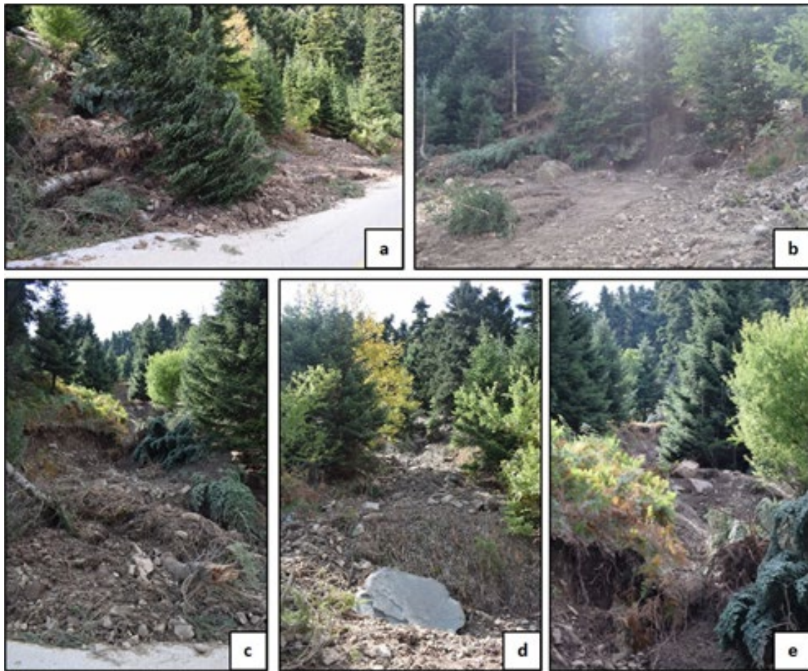
Figure 6.13. Rotational slide on the road to Oxya village (39.366667°N, 21.592222°E)
