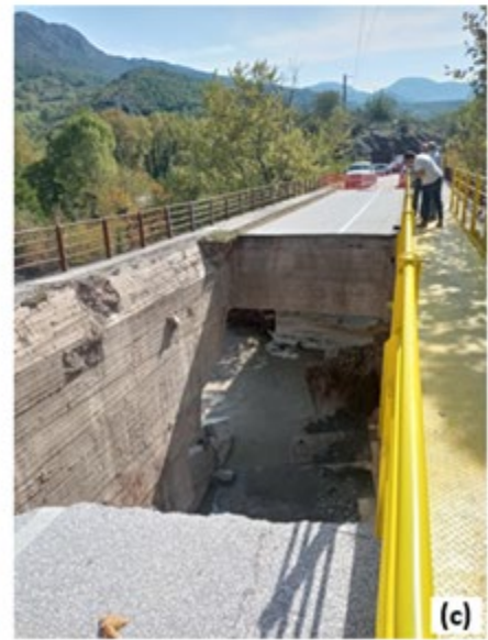
Figure 5.12. Photos of the collapsed Bridge No. 9 crossing Pamisos river about 2 km north of Mouzaki ( 39.406108333^{\circ}\text{N} ; 21.663150000^{\circ}\text{E} ): (a) side view indicating abutment backfill erosion and the location of the collapsed roadway segment; (b) closer view of failed abutment wall; and (c) the roadway gap.
