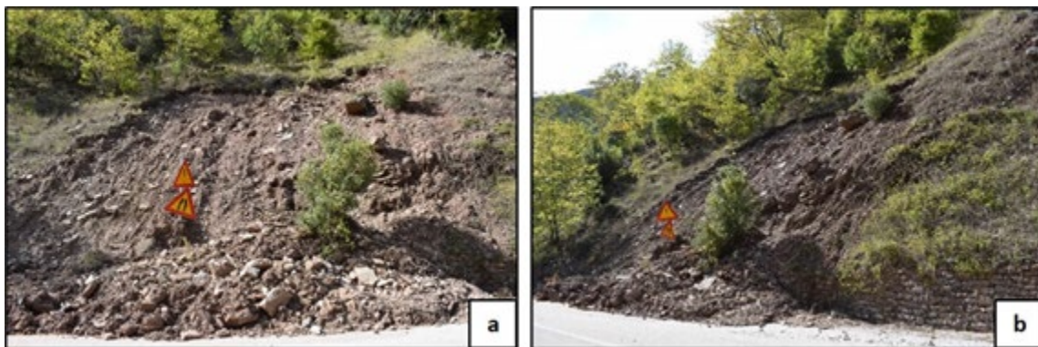
Figure 6.14. Rotational slide at Argitheia to Zervo road (39.351111°N, 21.521389°E).
