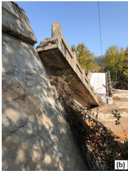
Figure 5.21. Photos of Bridge No. 11 ( 39.401172611^{\circ}\text{N} ; 21.652868250^{\circ}\text{E} ) which evidently collapsed due to a combination of abutment and pier scour: (a) side view, (b) - (c) bearing capacity failure of the abutment and deck collapse.
